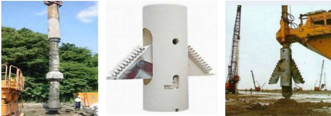
Fig. 1 Model of an under-reamed pile with a single full bulb [2].
