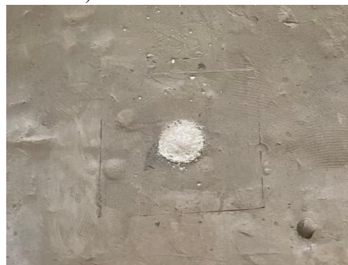
D) Completing the sand compaction process
