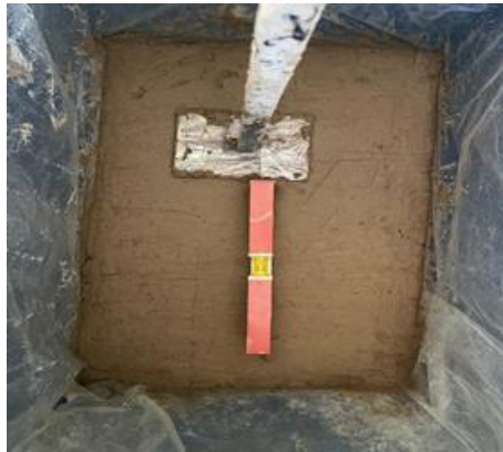
A) Soil compaction
